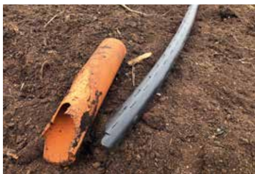
Figure 119. Ceramic and plastic pipes installed to establish a subsurface drainage system were found in Amalva. It is a legacy of the Soviet reclamation school from the late 1980s. Photo: N. Zableckis.
