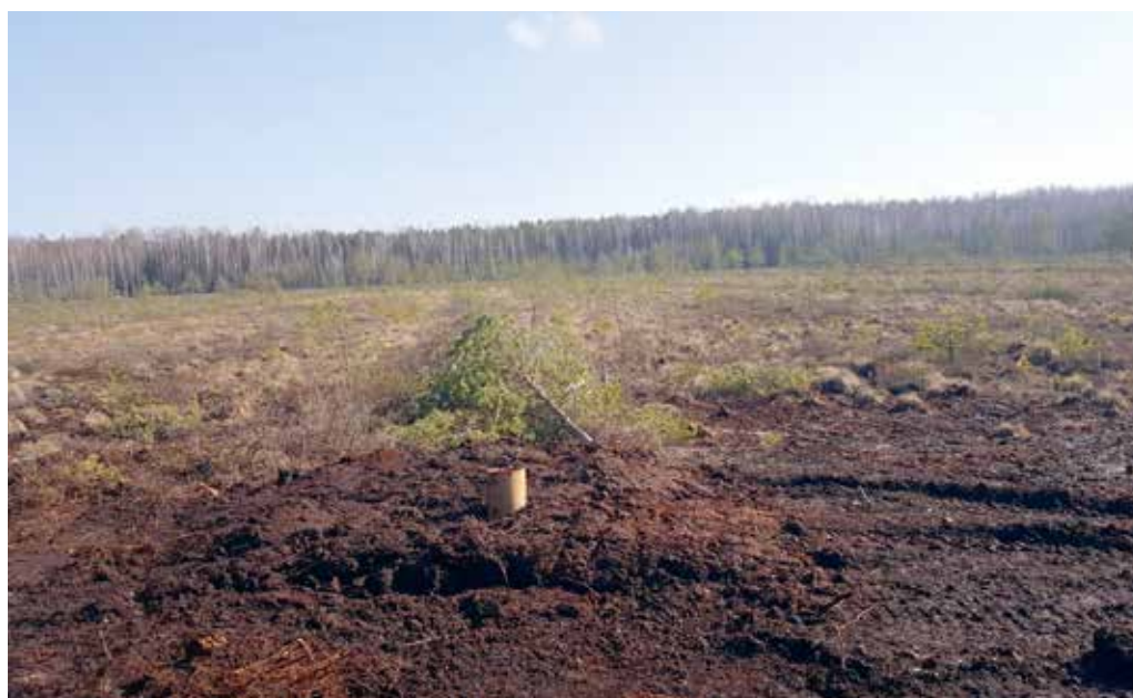
Figure 161. A peat dam located at the place where the old drainage pipe was broken, March 2020. Photo: L. Jarašius.
