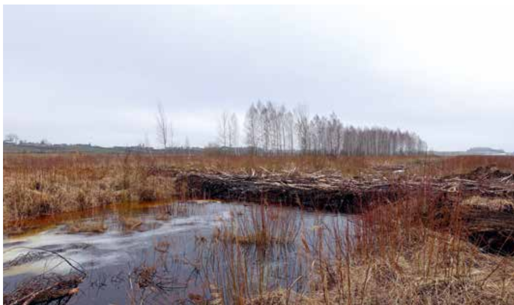
Figure 118. The blocked collective ditch in Amalva, March 2021. Photo: J. Sendžikaitė.
