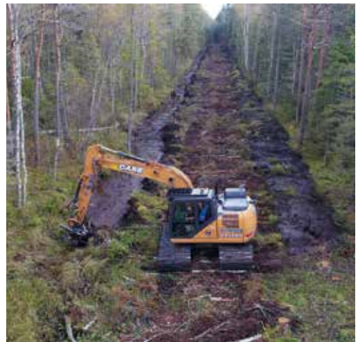
Figure 24. Opening of the old bed of Kaldemäe stream for fish migration. Photo: R. Pajula.
