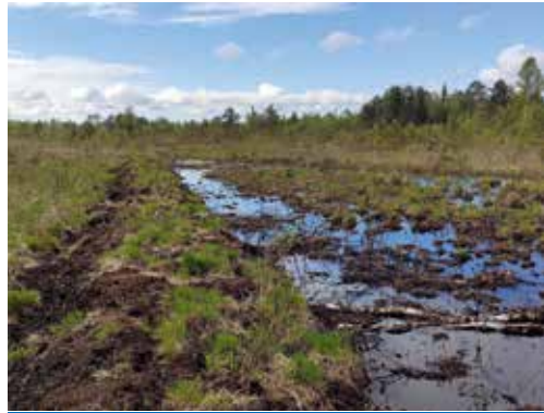
Figure 26. Raised water level behind the peat dike running along Piirsalu stream in spring 2021. Photo: R. Pajula.
