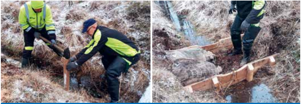
Figure 100. Manually built dams in Wielkie Bagno (winter 2021). Photos: W. Spychała.
