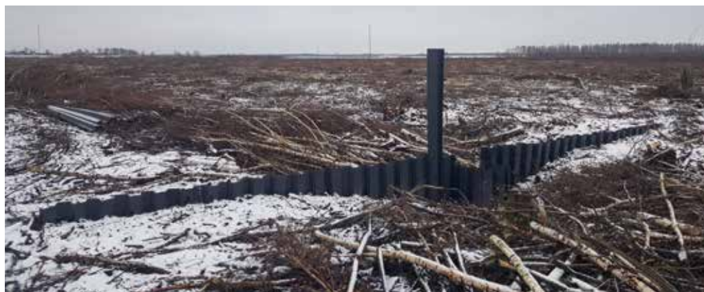
Figure 126. Installation of the plastic pile sheets dam. February 2021. Photo: Ž. Sinkevičius.
