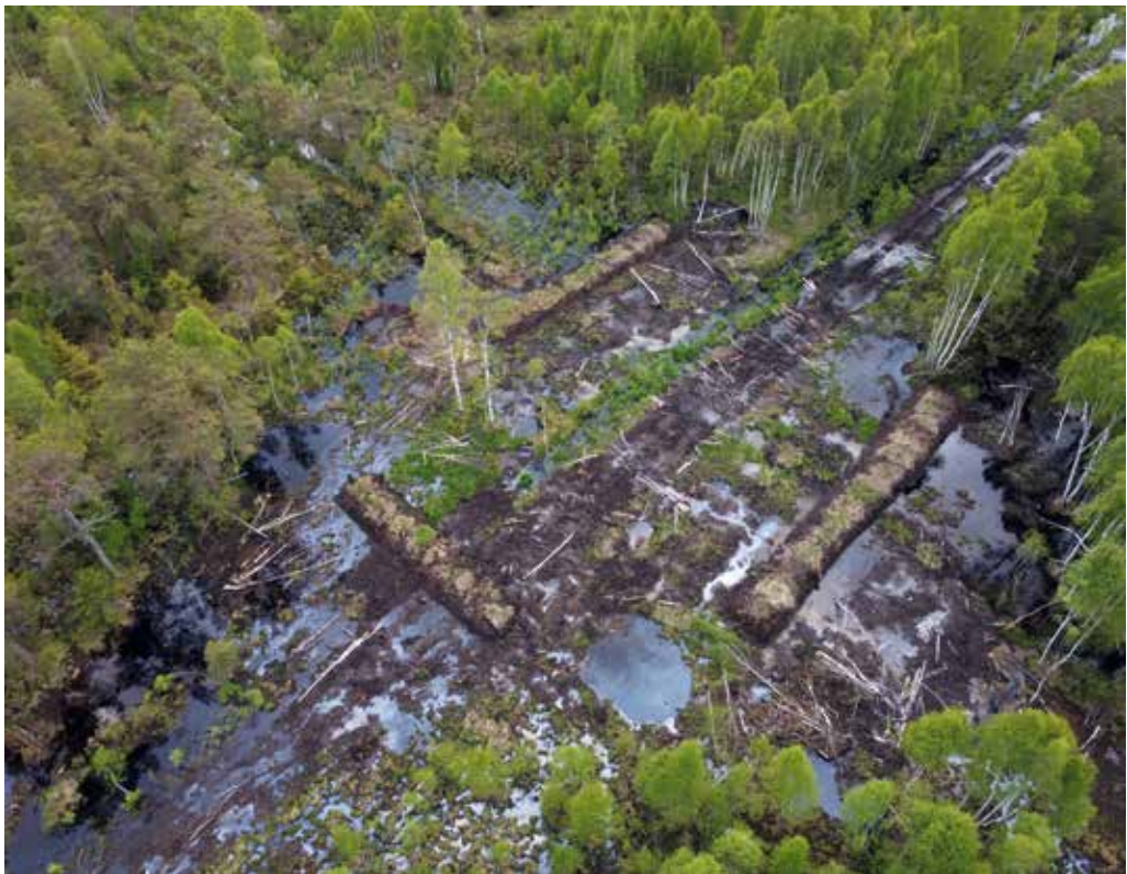
Figure 29. Aerial view of the ditch crossing in the eastern part of the Suursoo-Leidissoo restoration site in spring 2021 after the construction of the dams. The small pools are holes where peat was taken for dam building. Photo: R. Pajula.
