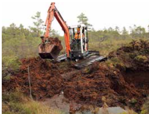
Figure 78. The excavator is building a peat dam. Photo: M. Pakalne.
