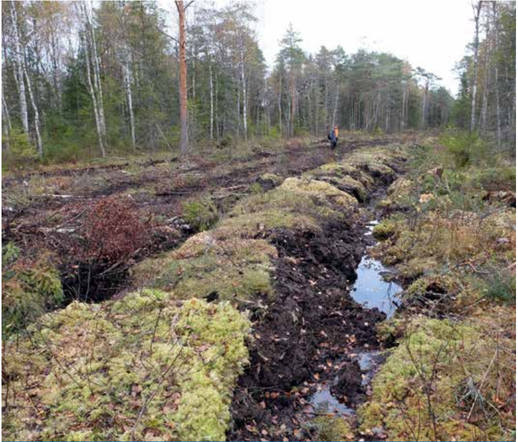
Figure 22. A peat dike built along the Kaldemäe stream, autumn 2020. Photo: R. Pajula.
