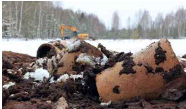
Figure 148. Old asbestos pipes were broken in order to restore water level in the Pūsčia peatland. Photo: J. Sendžikaitė.
