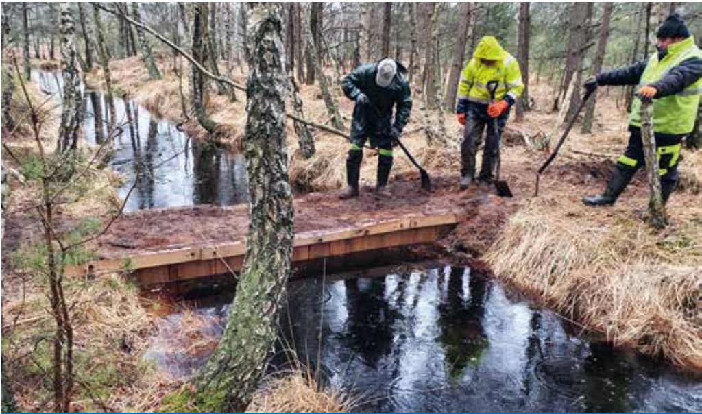
Figure 102. Dam building, March 2021. Photo: W. Sychała.
