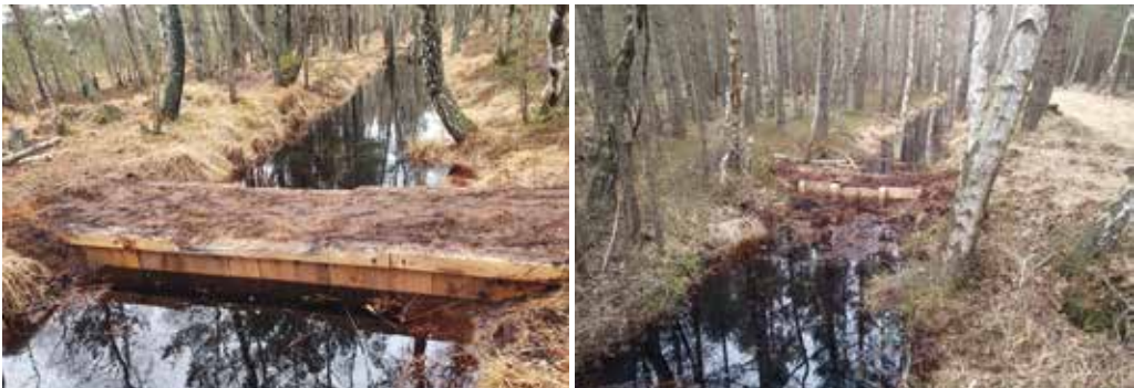
Figure 103. Examples of completed dams, March 2021. Photos: W. Sychała.
