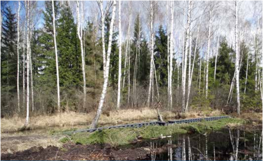
Figure 162. Plastic pile sheet dams were installed in particularly wet and difficult to access places, March 2020. Photo: J. Sendžikaitė.
