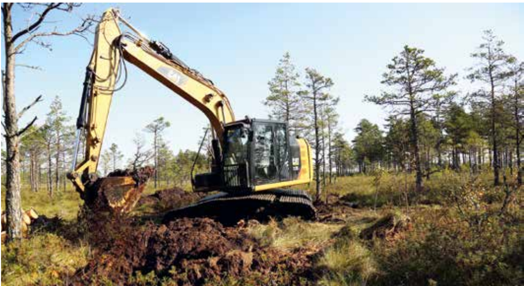
Figure 2. Building a peat dam by an excavator. Photo: M. Pakalne.
